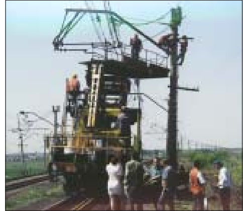
Fig. 11-26 Lashing optical fiber cable along a railroad. The cable is lashed to the neutral wire.
