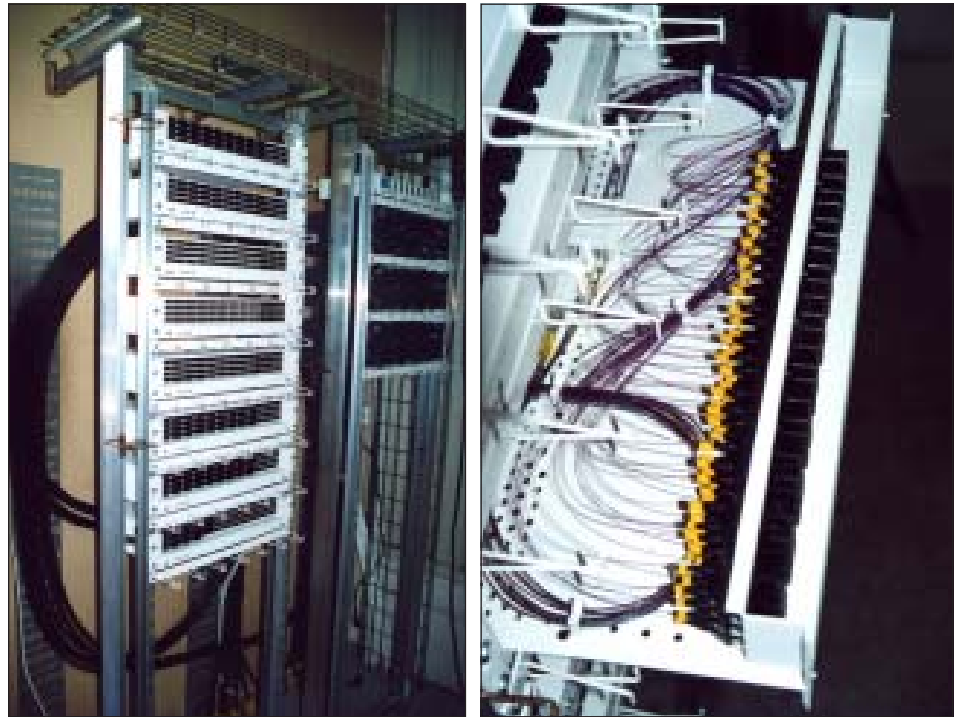
Fig. 11-50 and 11-51 To the left is a fiber distribution field that can accommodate 960 MTRJ connectors for fiber ribbon thus resulting in termination of 2 000 fibers or more. To the right is a termination unit with 96 connectors.
