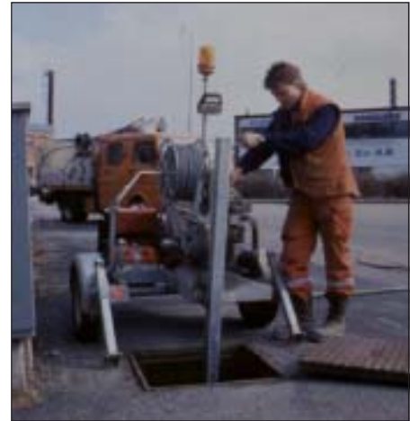
Fig. 11-13 Microprocessor-controlled winch for cable laying in ducts. (Photo, courtesy of Riteco AB)
