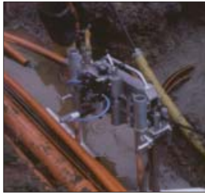
Fig 11-17 Floating with water, equipment set-up. Photo: Courtesy of Sahlins, Sweden
