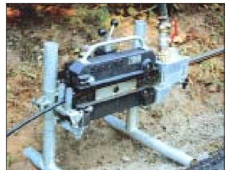
Fig 11-16 “Cable cat” in connection with compressed air equipment Photo: Courtesy of Sahlins, Sweden
