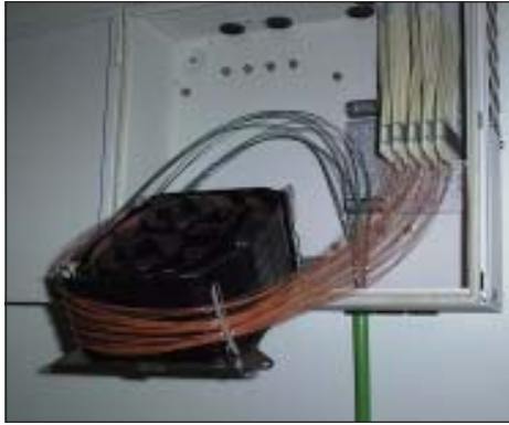
Fig. 11-35 Splice cabinet. 48 microducts are terminated and 48 2-fiber ribbons are spliced within the cassettes to the left. The green 96-fiber ribbon cable enters the cabinet at the bottom.
