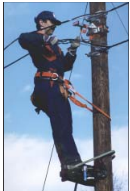
Fig. 11-21 Permanent fixing of the cables at the top of the pole.
