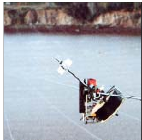
Fig. 11-27 Wrapping the optical cable around the high voltage power lines.
